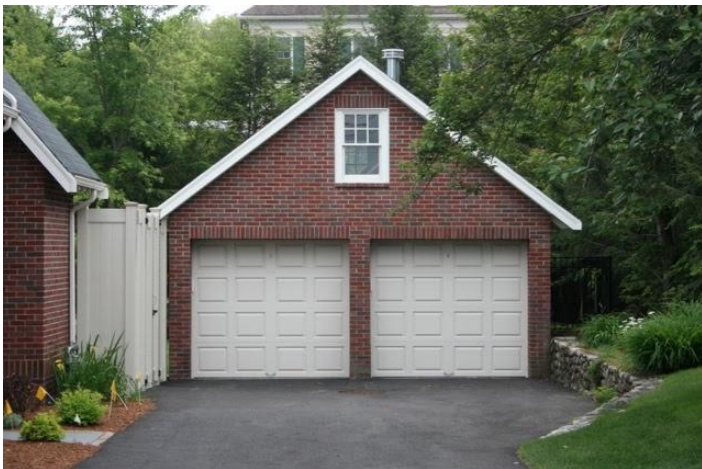
Garage: Front (facade) elevation
