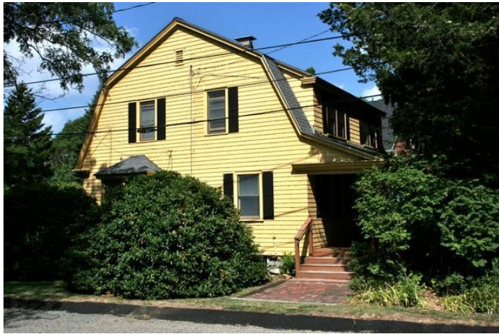
Left side (Balfour Street) and front (Asbury Street façade) elevations
