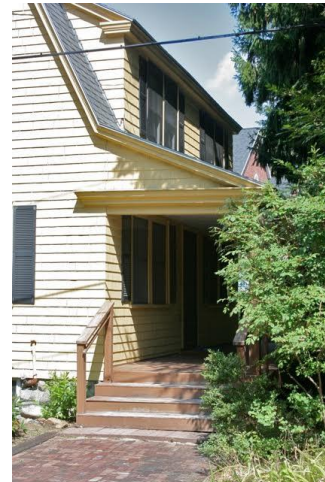
Front (Asbury Street façade) elevation: detail
