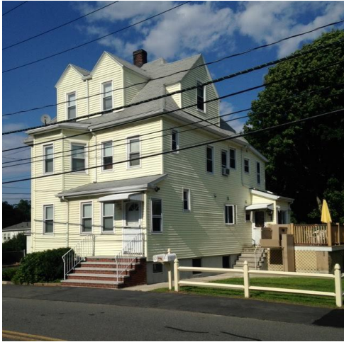
West (façade) and south elevations
