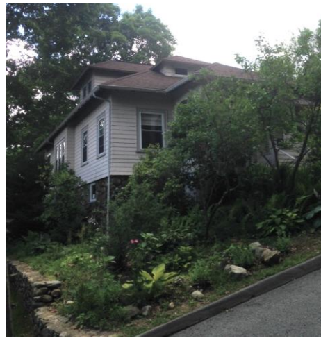
North (left side) and west (façade) elevations
