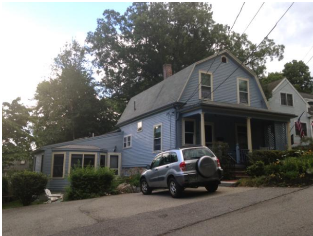
North (left side) and west (façade) elevations
