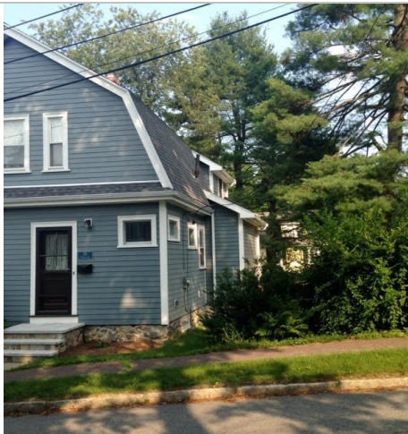
West (façade) and south elevations
