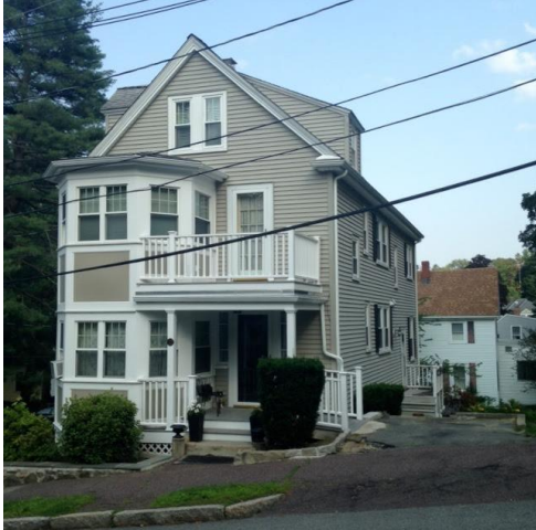
West (façade) and south elevations
