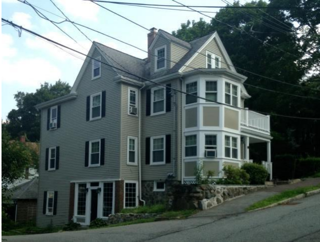
North (left side) and west (façade) elevations
