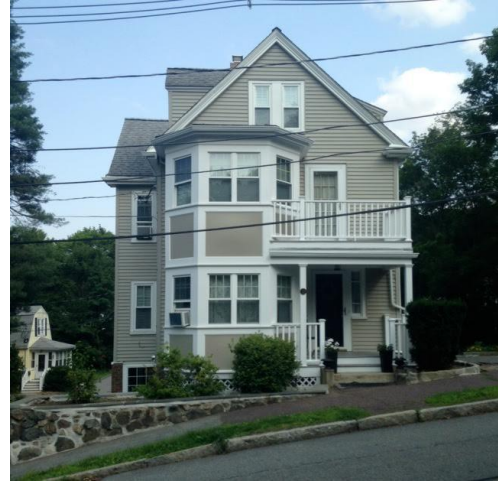
West (façade) elevation
