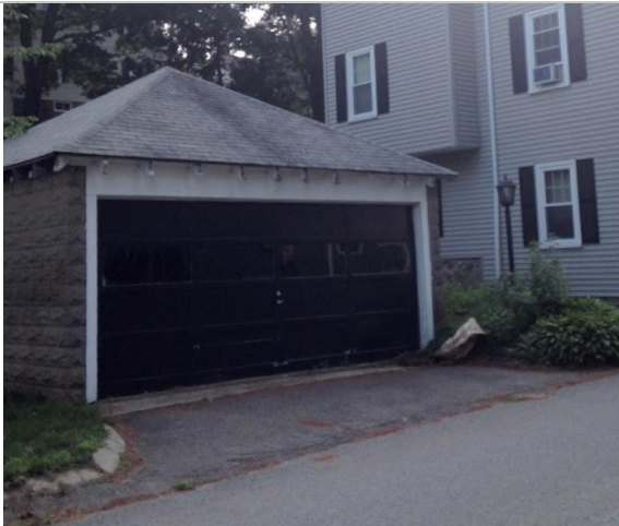
Garage: North (façade) elevation
