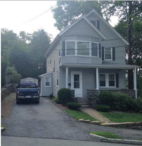
South (right side) and east (façade) elevations
