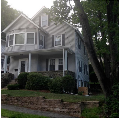
East (façade) and north (right side) elevations
