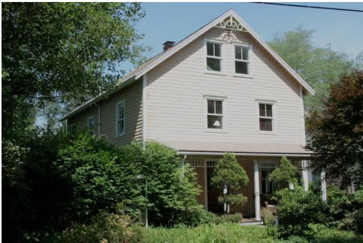
Left side and front (façade) elevations
