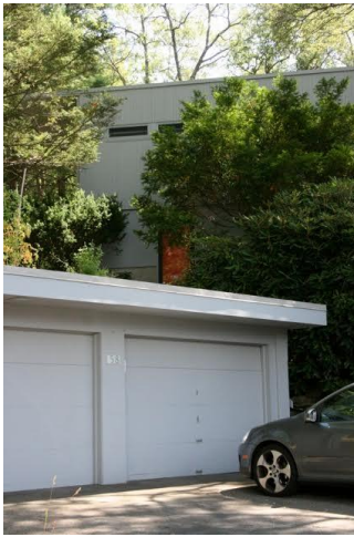
Front facades of garage and house
