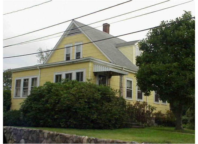
Assessor's photograph: Front (façade) elevation
