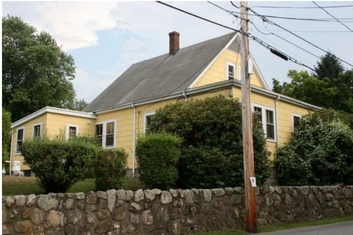
Left side and front (façade) elevations
