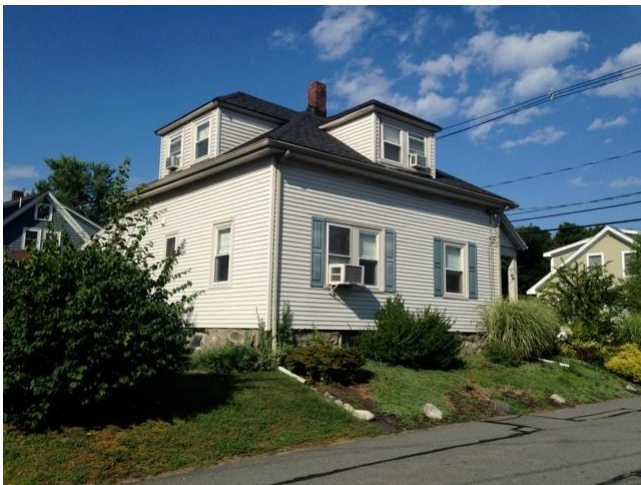
West (back) and south elevations
