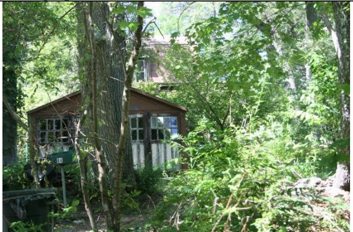
Garage and left side elevation of main house
