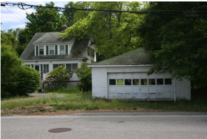
North (facade) elevations of house and garage
