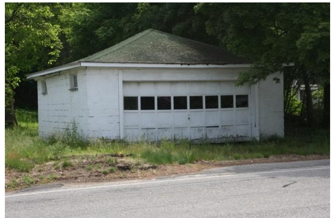
Garage: East and north (facade) elevation
