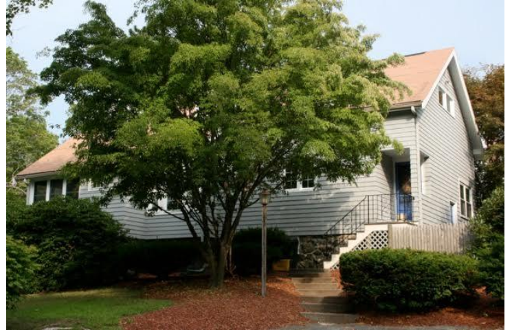
Right side (Kendall road) and rear elevations
