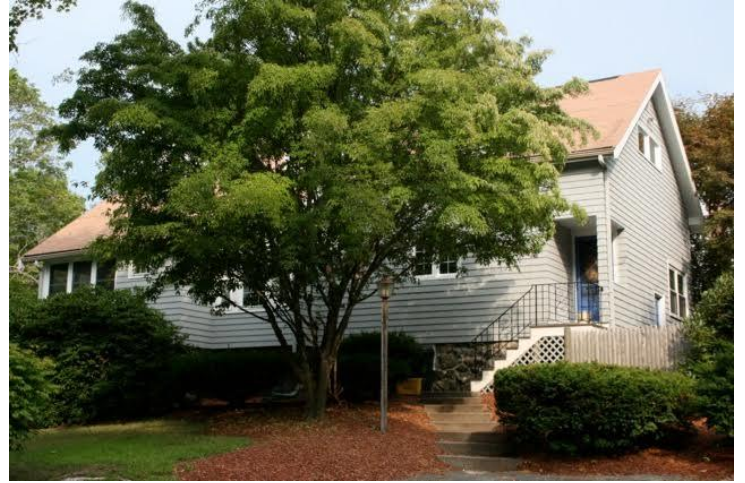
Right side (Kendall road) and rear elevations
