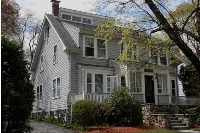
East and north (façade) elevations (view SW)
