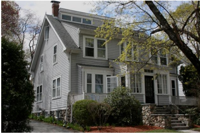
East and north (façade) elevations (view SW)
