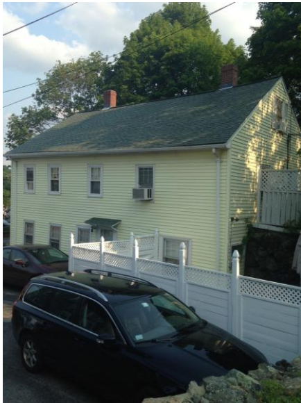
Right side (north) and rear (west) elevations
