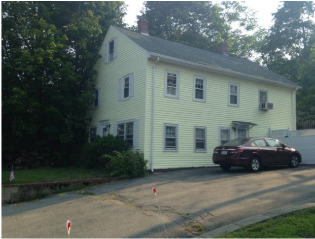
Front (east; Pleasant St.) and right side (north) elevations
