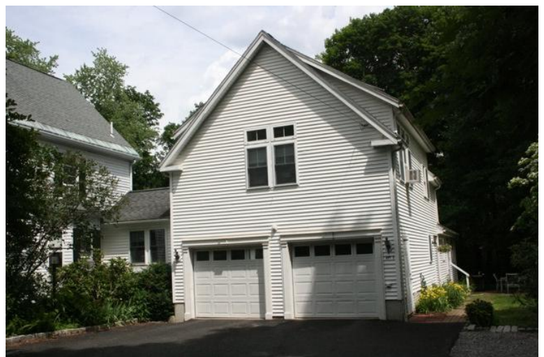
Barn: Front (facade) and right side elevations
