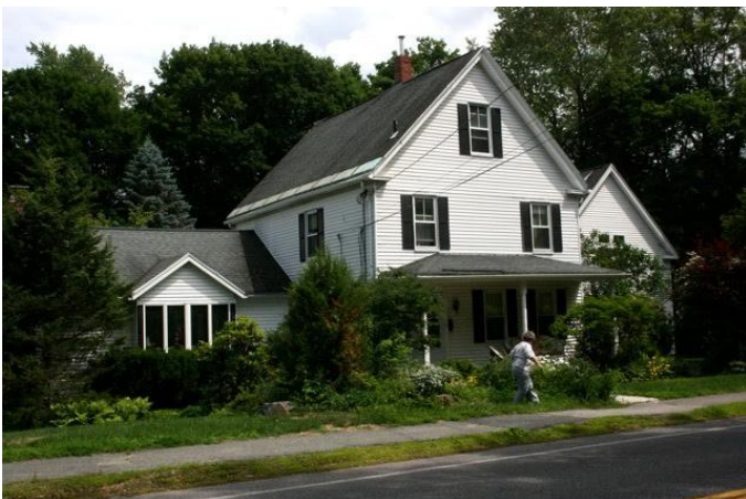
Left side and front (façade) elevations
