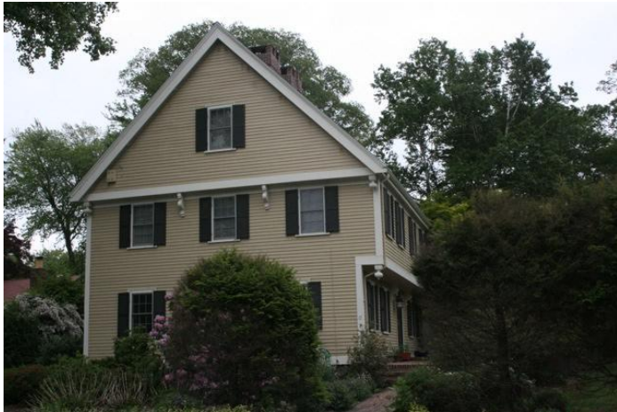
West and south (facade) elevations
