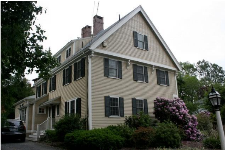
Back and left side (Hancock Street) elevations
