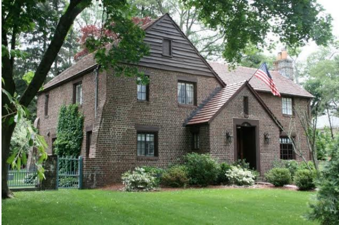
North and west (facade) elevations
