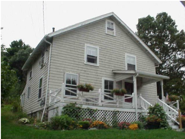
Assessors' photograph: South (left side) and east (façade) elevations
