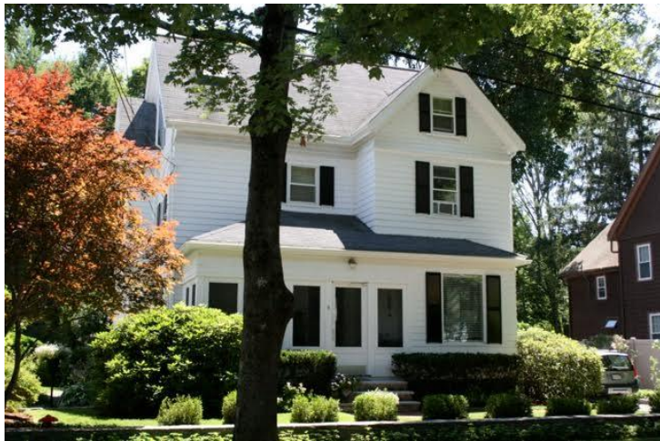
Left side and front (façade) elevations
