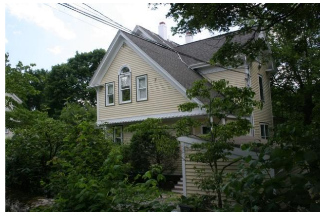
East and north elevations
