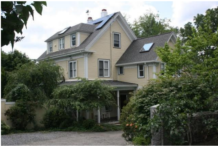
South and east elevations
