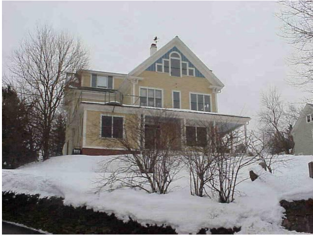
Assessors' photograph: West (facade) elevation
