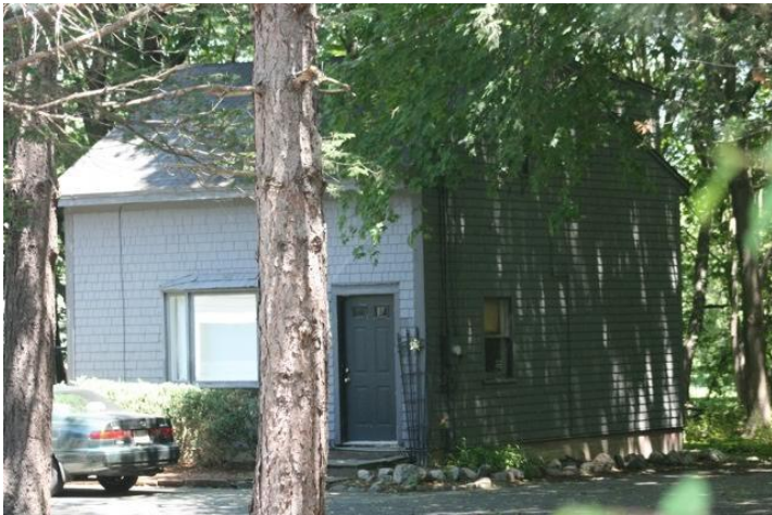
SE Outbuilding: West (facade) and south elevations
