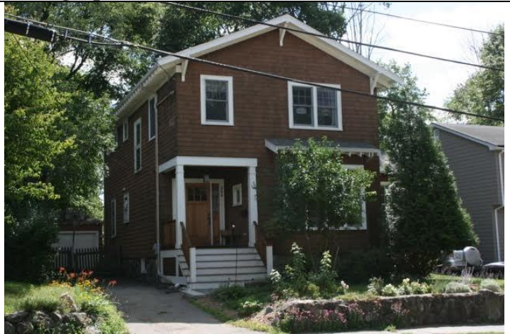
Left side and front (façade) elevations
