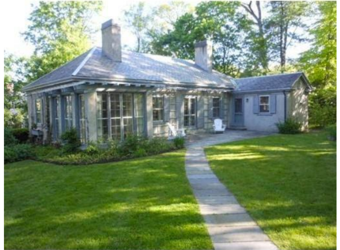
Original house: Front and right side elevations (Lester Savage photo, 2012)
