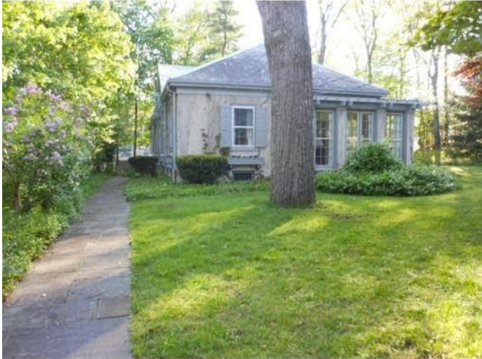
Original house: Front and left side elevations (Lester Savage photo, 2012)
