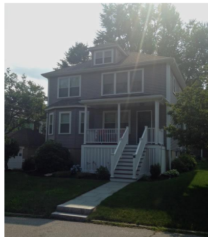
East (façade) elevation
