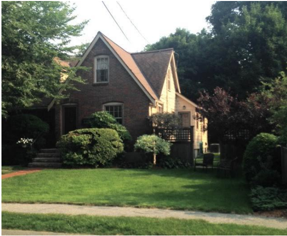
North (façade) and west elevations
