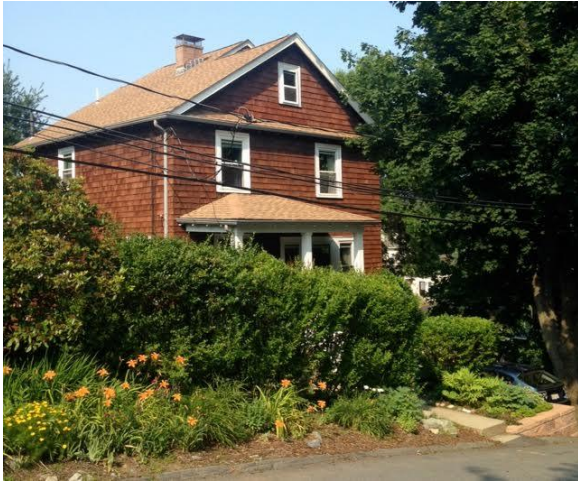
West (left side) and south (façade) elevations
